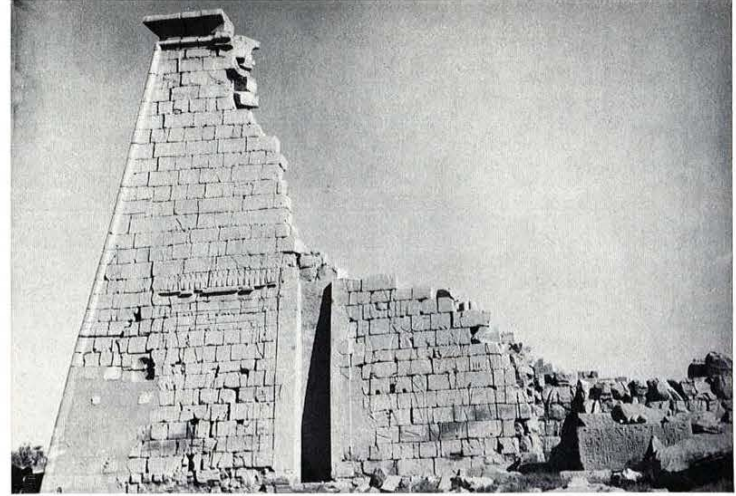
a) The western wing of Pylon IX before dismantling it
